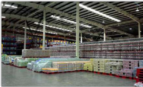
Coca Cola Mongolia Factory Lighting
